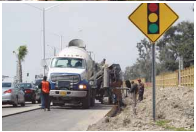
MDOT contractors install new curbing, part of the total remake of Beach Boulevard.
