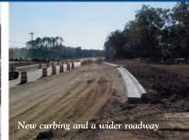
Laying material for a wider roadbed
