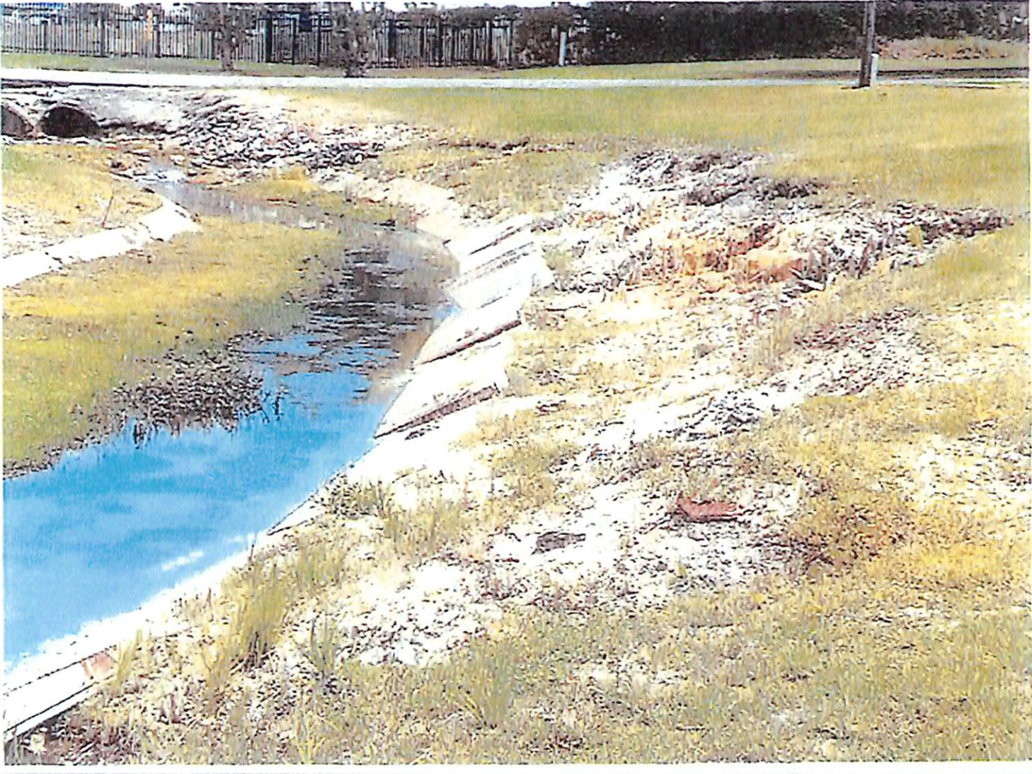
Hillier Park Nutrient Reduction and Storm water Control
