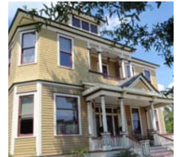
Restored Bond House, Biloxi
